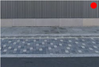
Mixed grey sett paving 100x200mm
