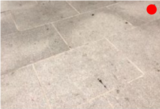
Grey granite flag paving 750x600mm
