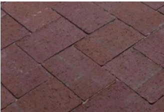
Clay brick paving 100x200mm (permeable where possible)
