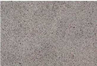
Insitu cast concrete paving with exposed brick aggregates
