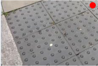
Charcoal grey blister tactile paving 400x400mm
