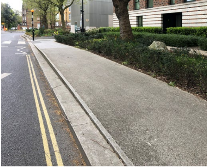
Example double-step kerb adjacent to existing trees at Elephant Park.
