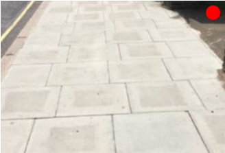
Grey concrete flag paving 750x600mm
